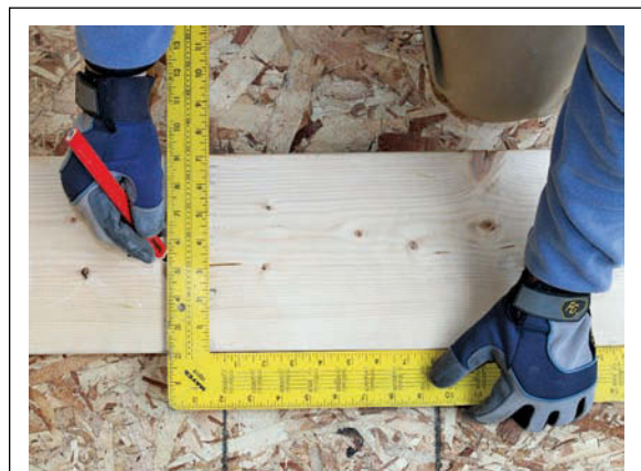
Figure 31 Marking a cutting line.
